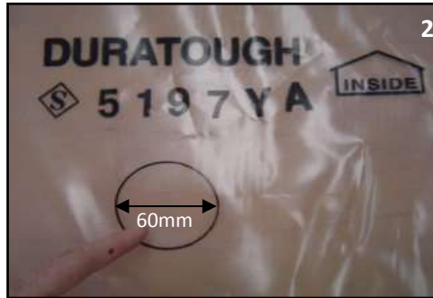
Mark a 60mm hole onto the inside twinskin cover at least 1 meter away from any of the films edges
