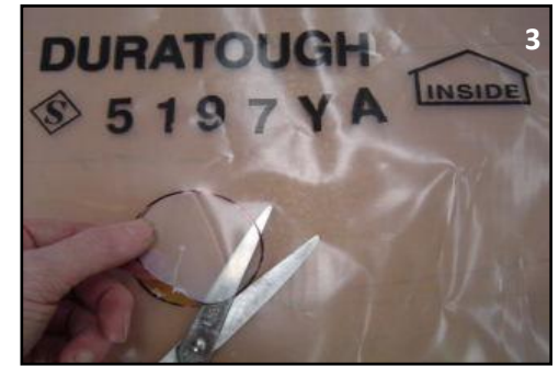
Cut out the 60mm hole, taking care not to accidentally cut the outer twinskin cover.
