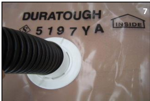
Plug in 65mm Air Pipe & ensure it "clicks" into the flanges internal locking lugs.
